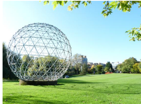
Figure 10: A 6m diameter aluminium dome, a gift from the British Aluminium Company on the occasion of the Third International Conference on Space Structures, University of Surrey, September 1984 [5].
