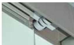
2 Sensors for detector of sash position
